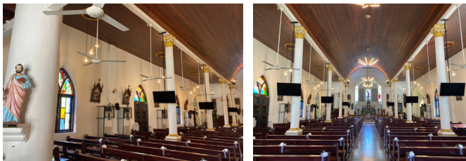
Figure 9 The interior of St. Peter's Church (Photographs by Lionel Thomas)
