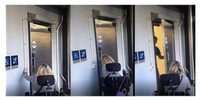
Figure 5 Broken switch access into the lecture room – student assistant required
