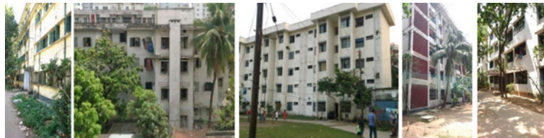
Figure 1 Azimpur, Green Road, Mirpur BCSIR, and Palashi Government Staff Housing (left to right) (Photographs by authors)
