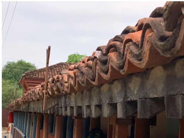
Figure 14 Texture of roof tile and weathered wooden members (Photograph by author)
